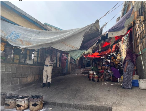
Figure 16: Plastic sheeting and textiles hung across pedestrian pathways and covering market stalls and transient workers; forming a bridge of combustible materials between buildings
