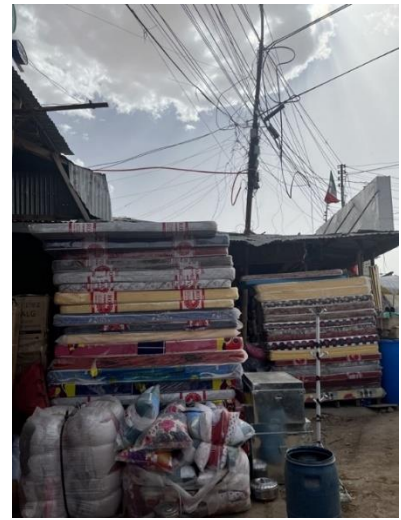
Figure 11: Combustible mattresses underneath electrical wires, including informal connections; Gobanimo Market
